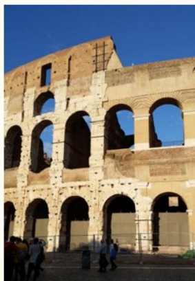
Figure 6: Old and new enclosures of the Colosseum.
